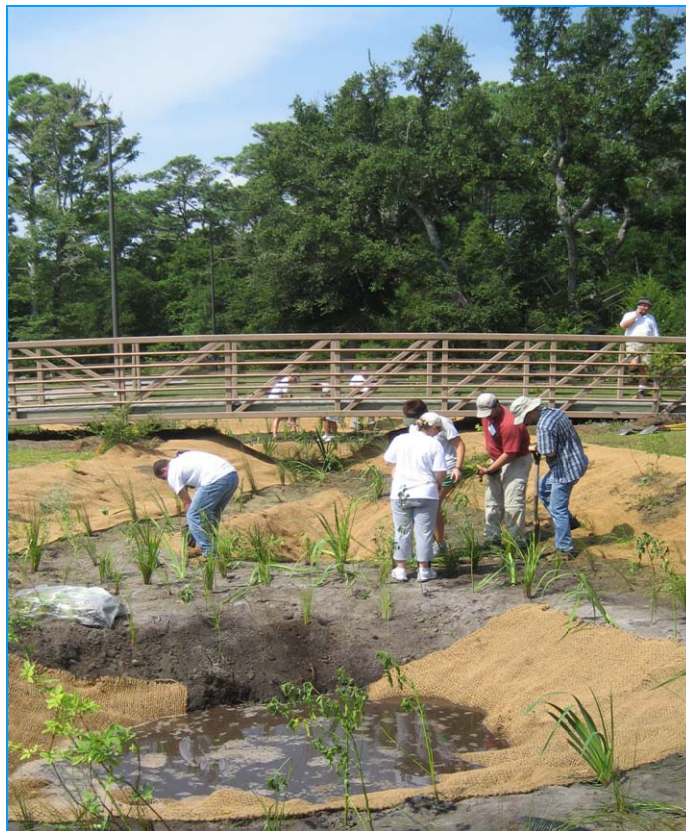
Stormwater Wetland Installation
